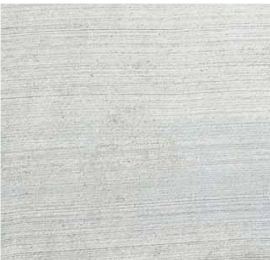
Concrete Paving with broom finish
